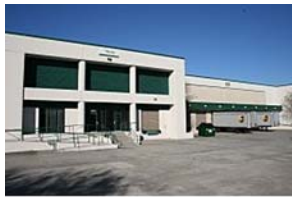
Silo Bend Dist Ctr 1
