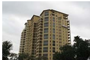
Bellamy on Bayshore
